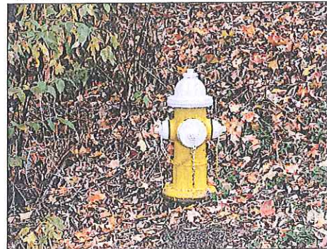
Water for Fire Protection Remains an Issue
