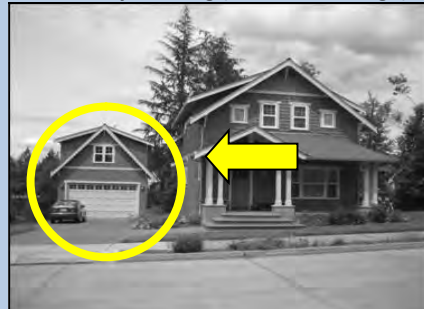
Accessory Building (Detached Garage)
