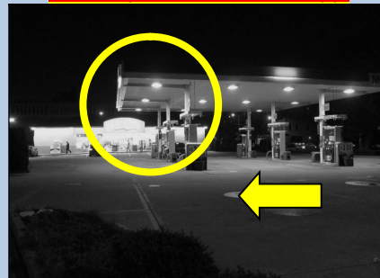
Accessory Structure (Gas Canopy)
