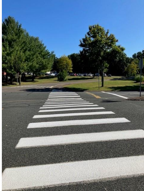
Vision Boulevard, crosswalk from elementary school driveway to maintenance facility driveway – needs ADA-complaint ramps
