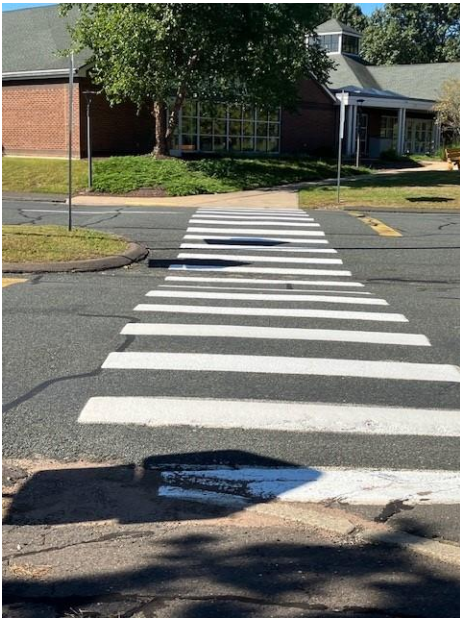
Vision Boulevard, crosswalk from middle school driveway to library – needs ADA-complaint ramps
